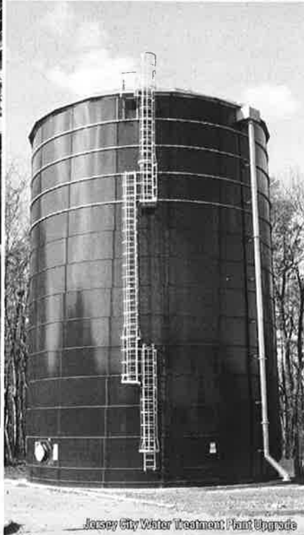
Jersey City Water Treatment Plant Upgrade
