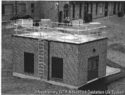
Neshaminy WTP Advanced Oxidation UV System
